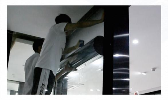
**Step 2.7:** Repeat the process (starting with step 2.5) until the installation is free of any air bubbles. Step 2.8 (below) should be paid close attention to, should air bubbles be trapped on the edges of the FILM.
